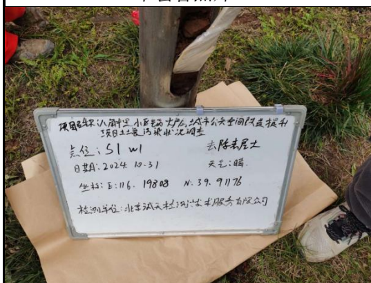
VOCs 取样-去除表层土
